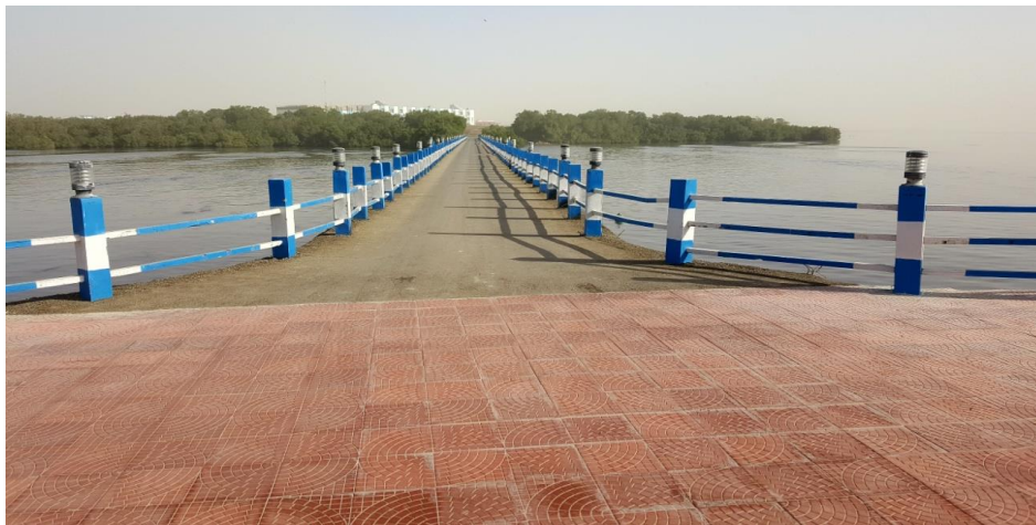
A BEAUTIFUL VIEW OF JETTY
